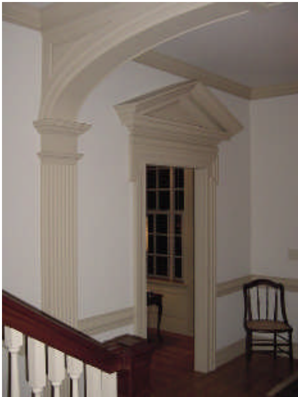
Millwork in the front entry hall.
